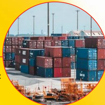
Doha, Qatar Integrated port infrastructure
